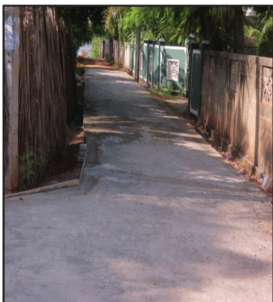
Concreting the road in Merawala Harinda area ((Length 52 m)
