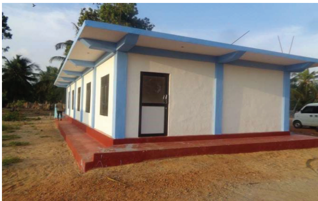
Renovation of Wannimundalama Multipurpose Building
