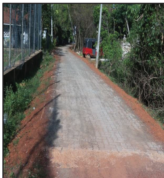
Concreting the road commencing from the volleyball court at first lane in Merawala colony. ((Length116 m)
