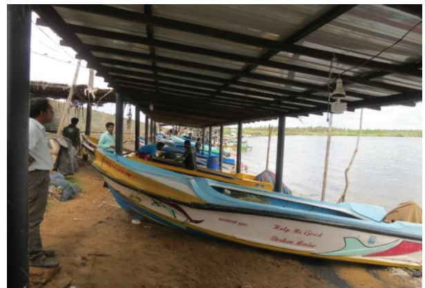
Construction of light shades at Kallukullia
