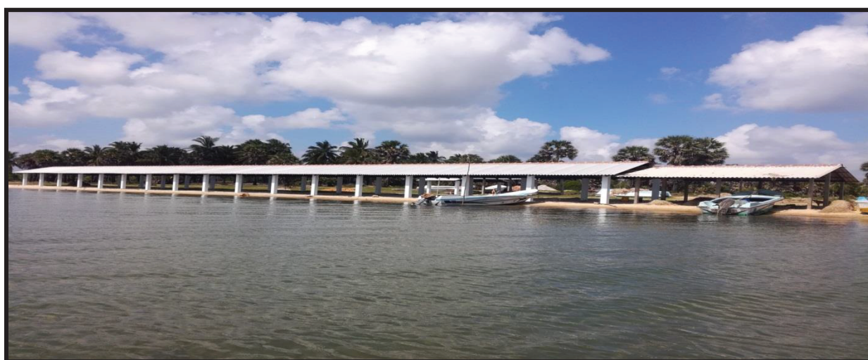
Construction of an open shed for parking boats
