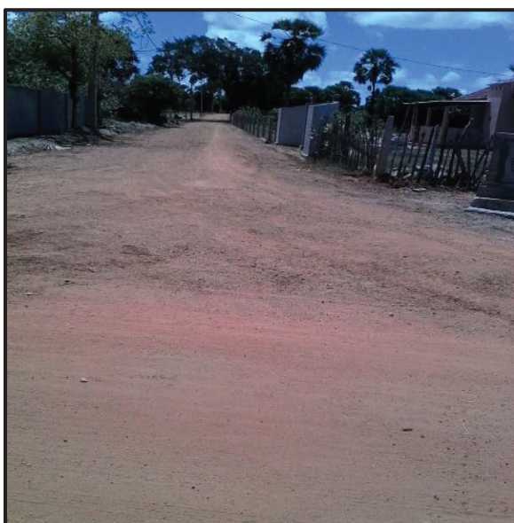
Tarring the public building road
