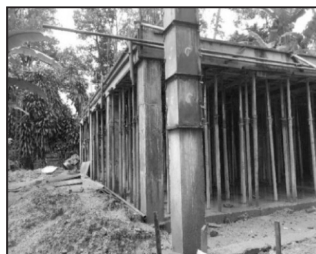
Construction at Haliela Veterinary Surgeon's office
