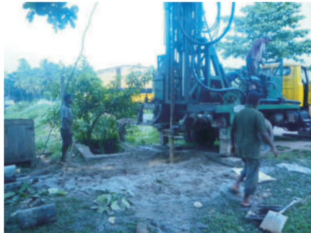
Test well construction at Biyagama
