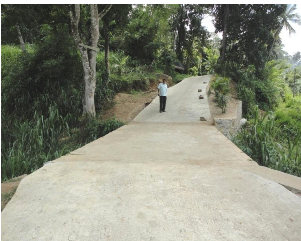
Agri Road Eramudugoda, Haloluwa and bridge
