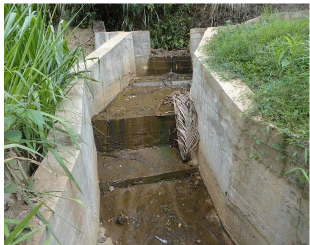
Construction of kohowiladeniya Anicut - Galagedera
