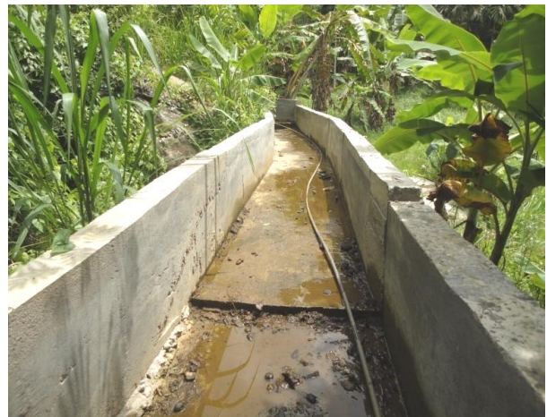
Construction or irrigation canal-Aralupota- Harispaththuwa
