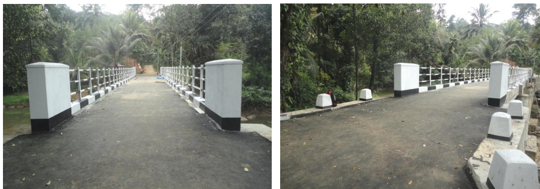
Viwala Bridge – Hataraliyaddha
