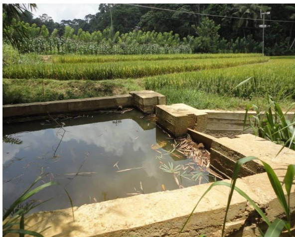
Canal bund renovation Vinguhumpola Galamuna Field Harispattuwa
