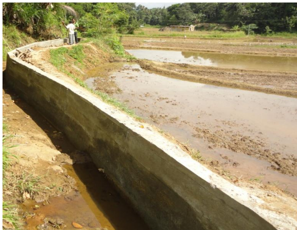
Retaining Wall – Kumbuka Paddy Field
