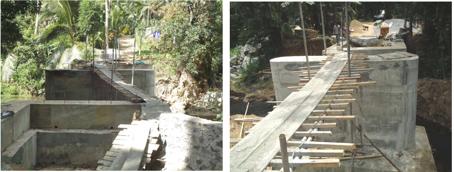
Narangaspitiya Vewala bridge which is under construction
