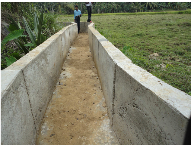
Harispattuwa, Malagammana Akkurawatta, Irrigation canel.
