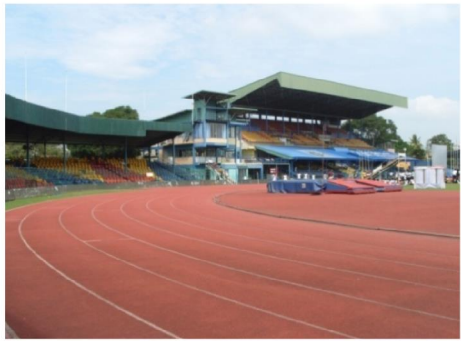
400 meter synthetic running track and the play ground
