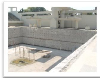
Diving pool repair works in progress
