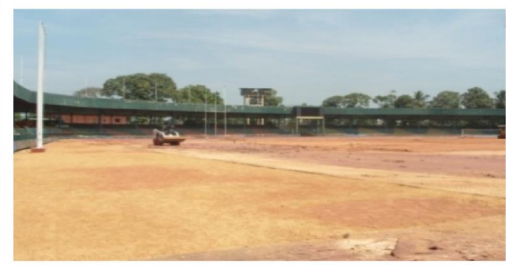
The 400 meter synthetic running track and the play ground under renovation
