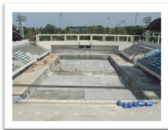
Main swimming pool repair works in progress
