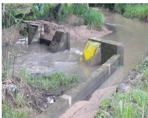
Construction of Pahatha Arawa Amuna of Siyambalanduwa
