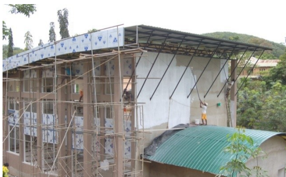
Fig. 9. Construction of Auditorium in Progress
