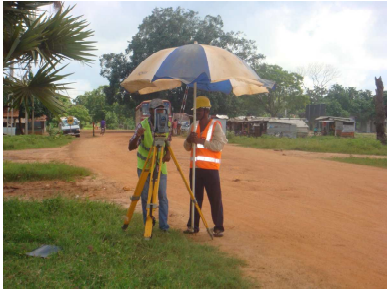
Continuing Survey Works
