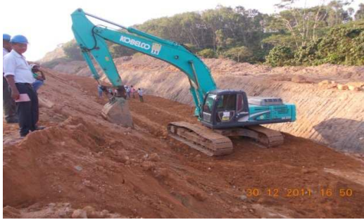
Embankment Filling at Ch. 43+700 – 43+ 850
