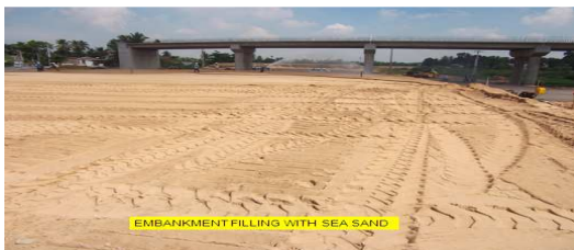
Embankment Filling with Sea Sand
