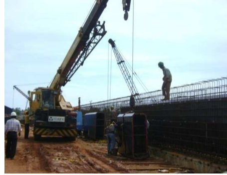
Inner shutter fixing for beam
