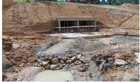
Preparation for fixing of Dowel Bars to RCBC Extension at Ch. 45+340
