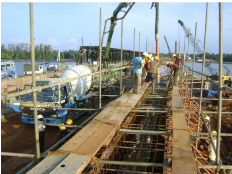
Concreting work for Beam
