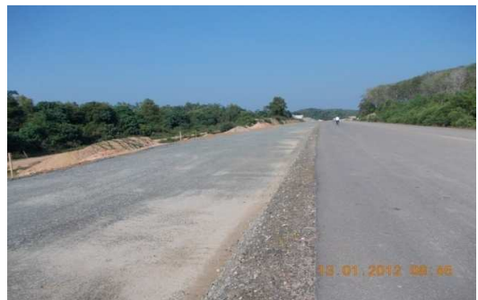
Laying of Sub Base 1st Layer at Ch. 54+320 – 54+780
