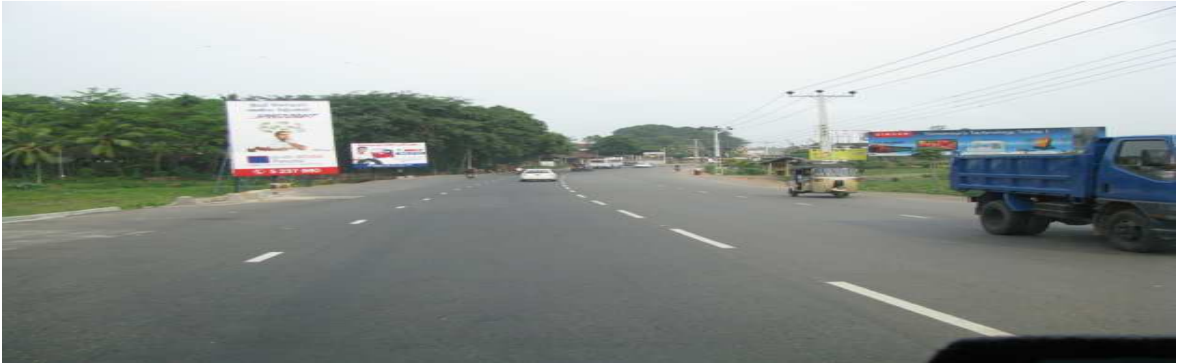
Road Section at 12+500 km
