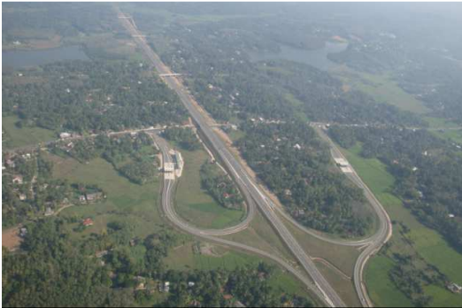
Arial View of Gelanigama Interchange
