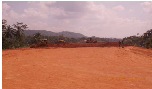
Embankment Preparation at Ch. 32+400~32+520
