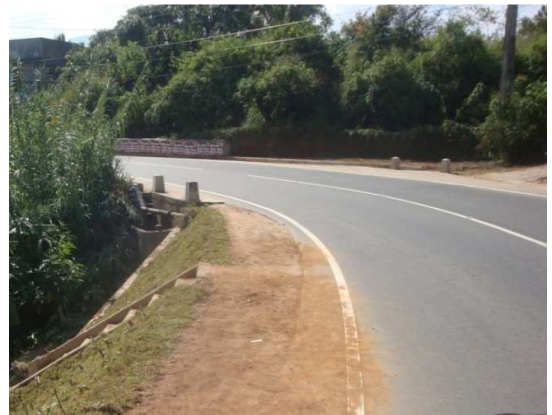
Turfing on embankment slope at 92+700km, LHS
