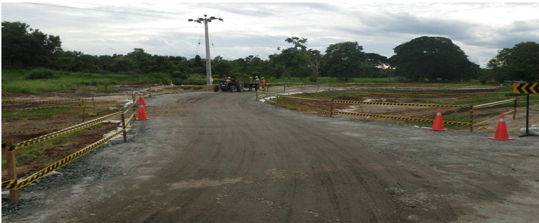
Bridge No 3- Detour construction completed
