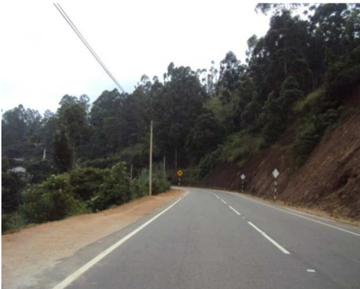
Finished road surface at 88+550 km
