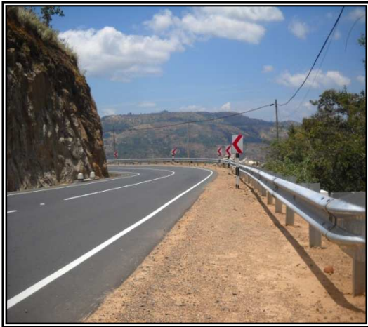
Crash Barrier at 40+700 km
