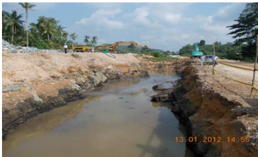
Unsuitable soil excavation at Ch. 50+800 – 50+860
