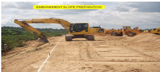
Embankment Slope Preparation
