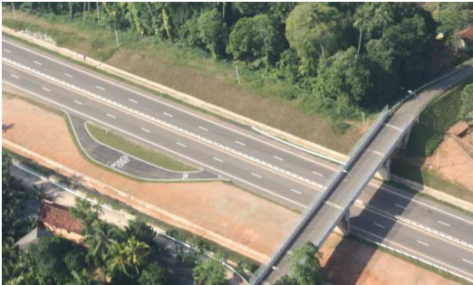
Arial View of Police Parking area and Overpass Bridge
