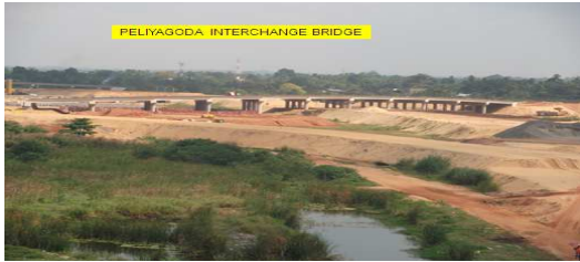
Peliyagoda Interchange Bridge
