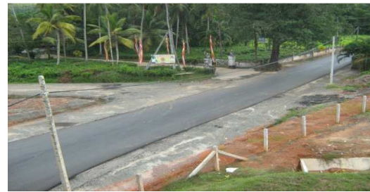
Asphalt Laying at UB 3 Diversion Road
