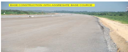
Base Construction with Aggregate Base Course
