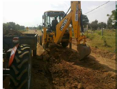
Widening for EW Filling 0-5km Section - Paranthan
