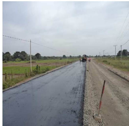
Kandy – Jaffna Road Ch. 209 + 700 km
