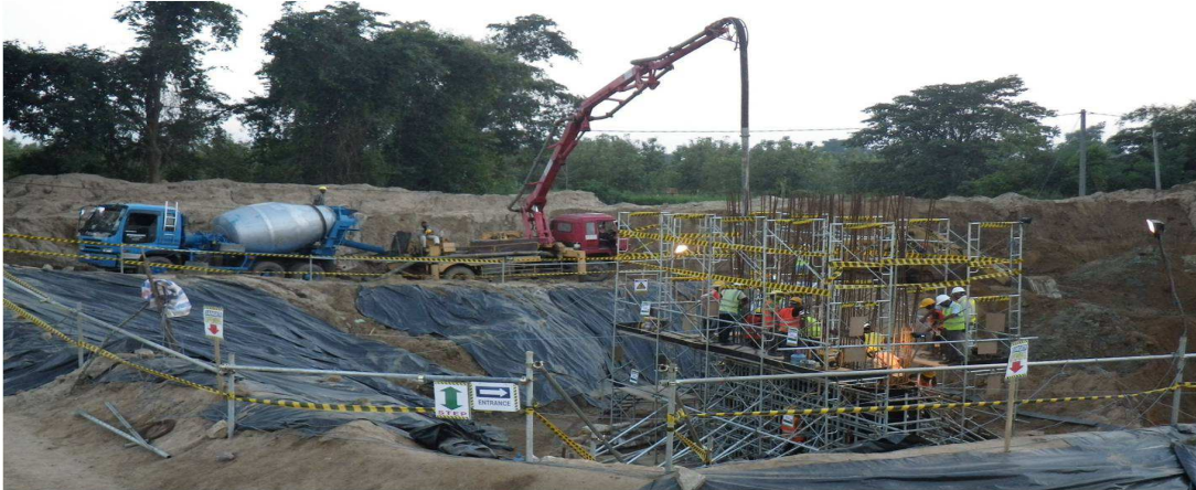
Placing concrete – Bridge No 1 Pier construction
