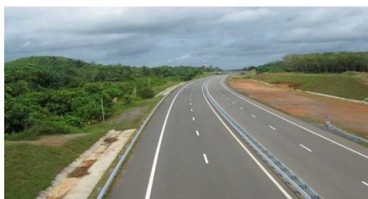
North View from Ch 37+500
