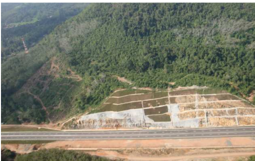
Arial View of Cut area at 29 km
