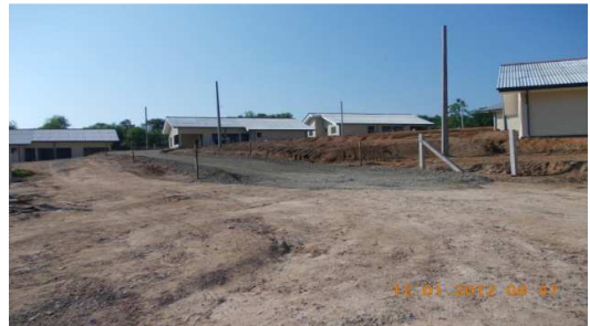
Construction of Engineer's Accommodation at Ch. 54+200
