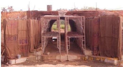
Curing of Concrete wing wall of RCBU Extension Ch. 31+007
