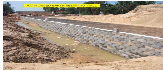
Reinforced earth Retaining Wall
