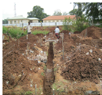
Eng's House Construction Started – Mankulam
