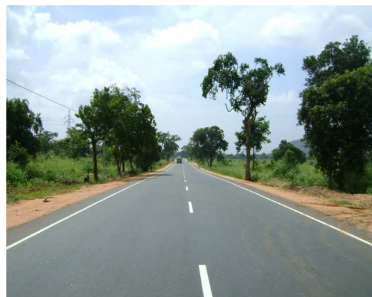
Road Marking Completed Section at 6 th km
