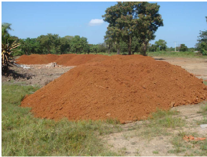
Stockpiling of Embankment Fill Started – Paranthan
