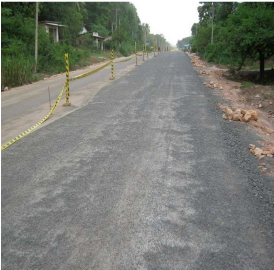
Kandy – Mahiyangana – Padiyathalawa Road Ch. 74+000 – 74+500 km
