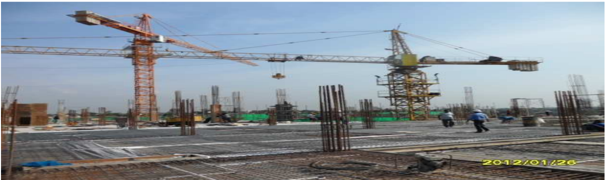
Structural work at Level 7- 8
