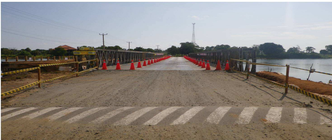
Bridge No 5 – Detour construction completed
