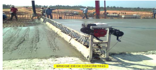
Bridge deck Concreting
