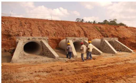
RCP Drainage End Section Construction at Ch. 32+754
