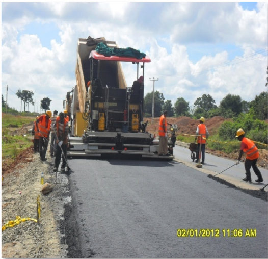
Kandy – Jaffna Road Ch. 263 + 600 km
