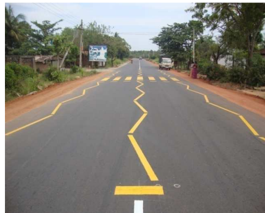
Completed road section at 58+580 km
