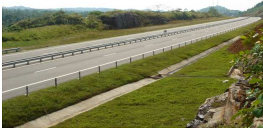
Ch. 1+600 Facing South
