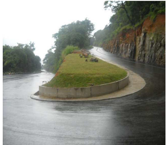
Completed binder course, 7th hairpin bend at 58+580 km
