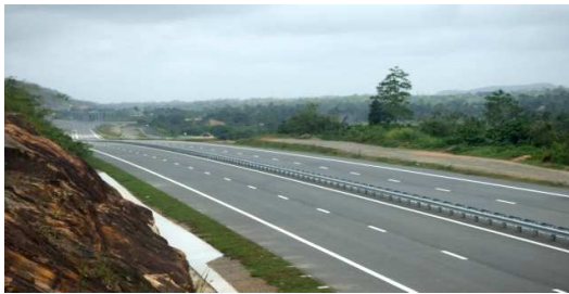
Median WRSB installation
