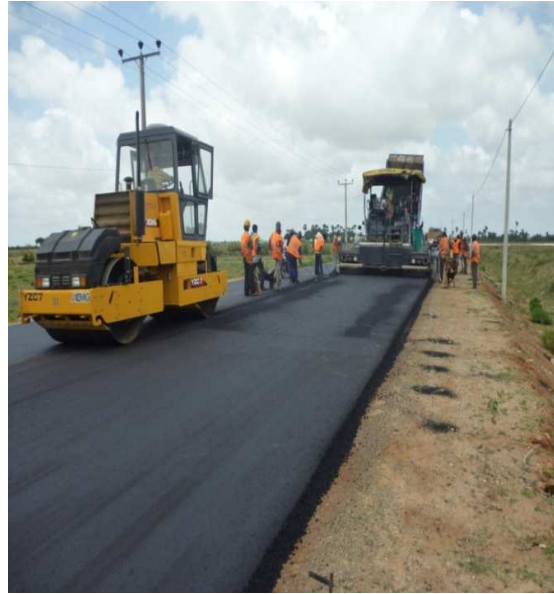
Jaffna Point Pedro Road AB020 – Ch. 23+750 km
