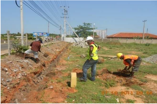
Excavation for parapet walls
