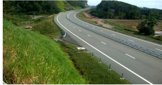
Ch. 18+500 Facing South
