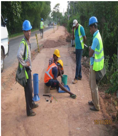
Mahiyangana – Dimbulagala – Dalukkane Road (0.0 -24.10 km)
