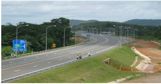
North View from Ch 47+000
