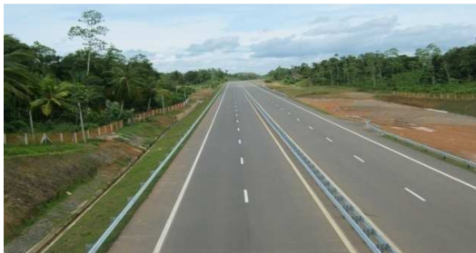
North View from Ch 55+600
