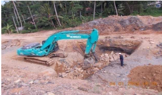
Soft Ground Treatment at Ch. 44+112
