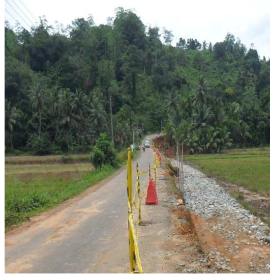
Pelawatta – Kankotiyawatta – Thiniyawala – Morawaka Road Ch. 2+500 km
