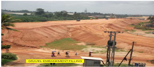
Gravel Embankment Filling
