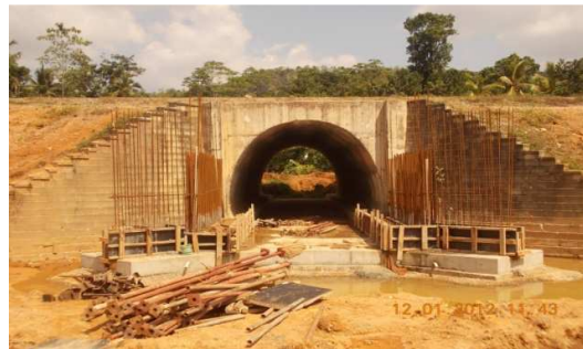
Reinforcement for RCBU Extension at Ch. 35+090
