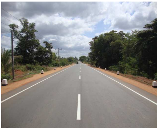
Completed road section at 39+308 km
