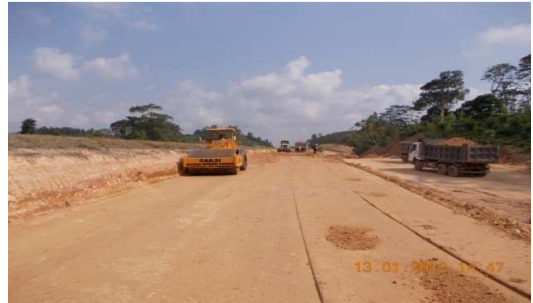
Embankment Filling at Ch. 52+775 – 52+850
