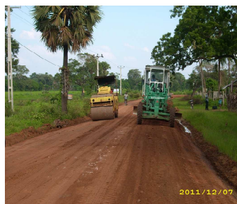
Initial Road Maintenance
