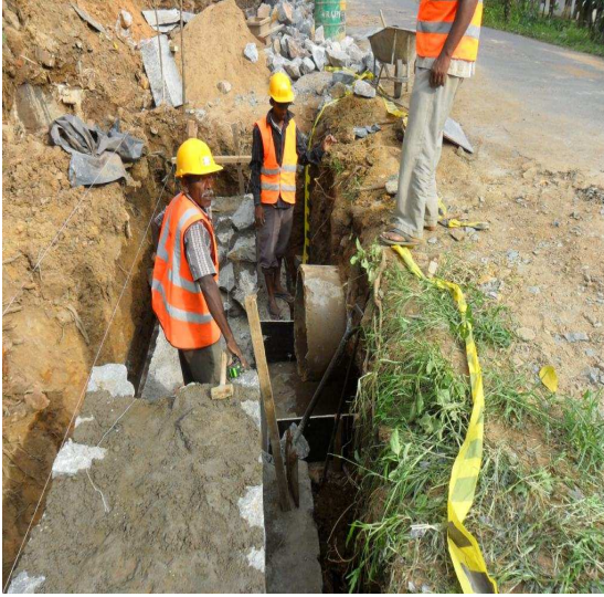
Pelawatta – Kankotiyawatta – Thiniyawala – Morawaka Road Ch. 1+130 km
