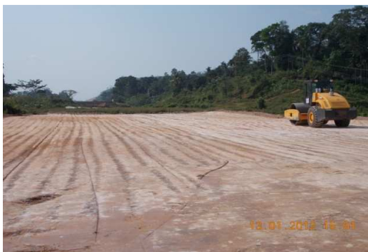
Embankment Filling at Ch. 50+650 – 50+780
