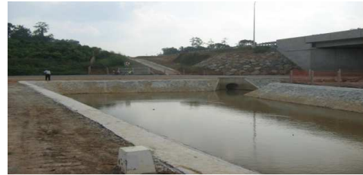
Construction of Water Pond Completed at Ch. 62+400
