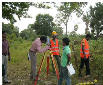
Topo Survey in Progress ( 0 – 5km)
