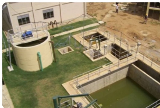
Sludge handling area of Hambanthota WTP
