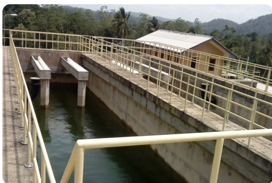
Sedimentation Tank of Akuressa WSS
