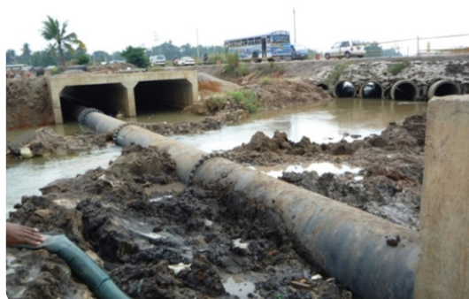
Re-routing of N33 Main at Makumbura
