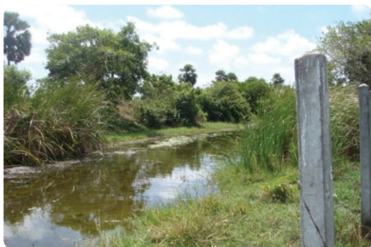
Murunkan Well Field - Source for Mannar WS and starting point of new raw water transmission main from Verugal River
