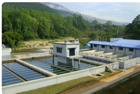
Meewathura Water Treatment Plant
