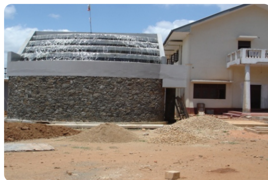
Aerator of Ipalogama WSS
