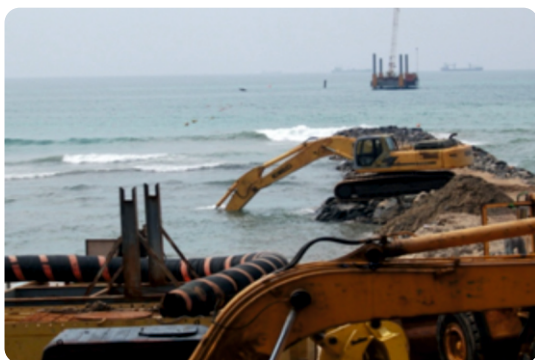
Construction of Sea Outfall near Lunawa Lagoon
