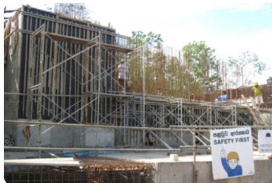
Construction of Ground Sump of Kirindi Oya WSP
