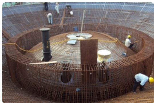
Construction of Kesbewa Water Tower
