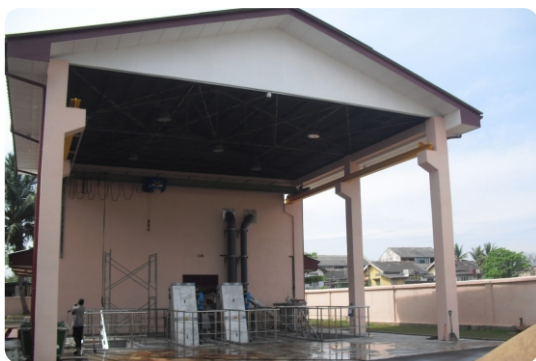
Completed Wellawatte Sewerage Pump Station
