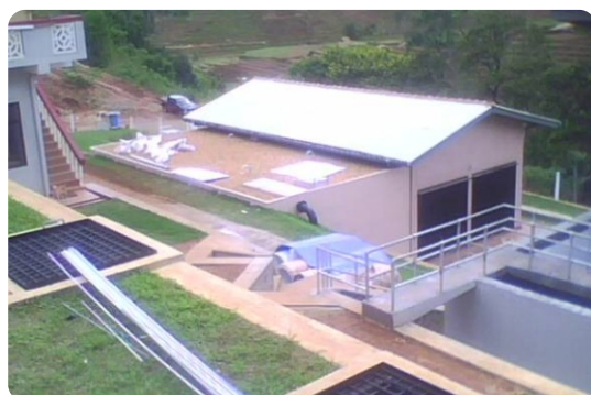
Part of the Ohiya WTP
