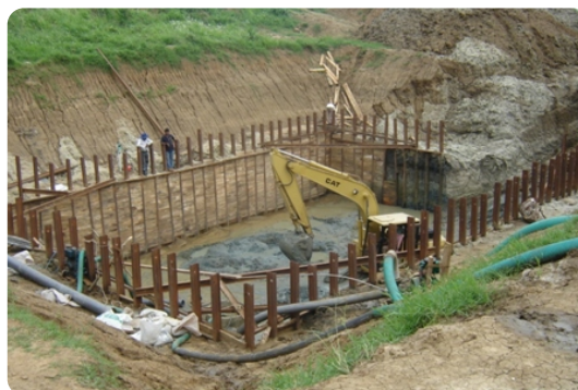
Construction of new intake at Allai Kantale
