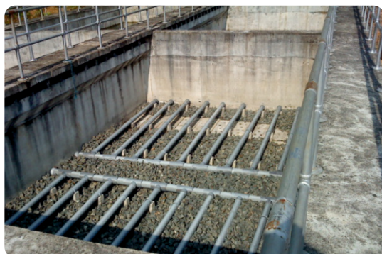
Rough Filter of the Udugama WSS
