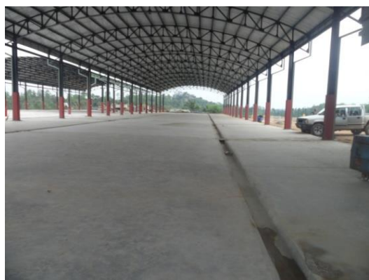
Completed undercover yard
