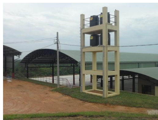
Completed Water Tank & undercover Yard
