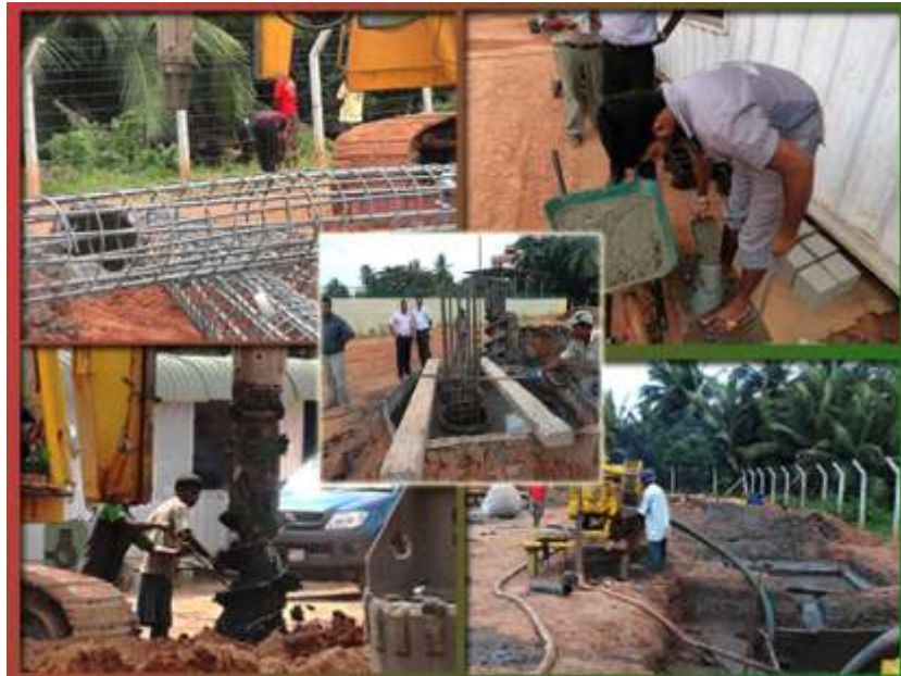
Fig: 5.6 Work In Progress at the NDT Site
