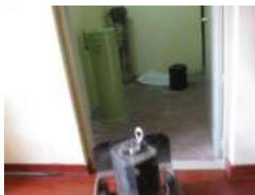
Fig: 2.2 Central Waste Storage Facility at AEA
