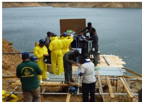
Fig No.20: Pumping set-up
