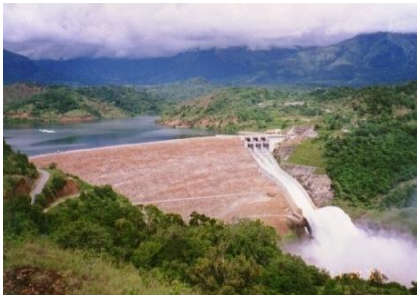
Fig No.17: Samanalawewa Dam
