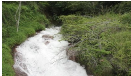
Fig No. 18: Amount of leakage -2.5 m 3 /S
