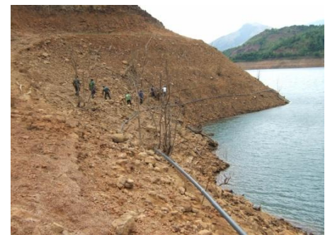
Fig No. 21: Pipes laid
