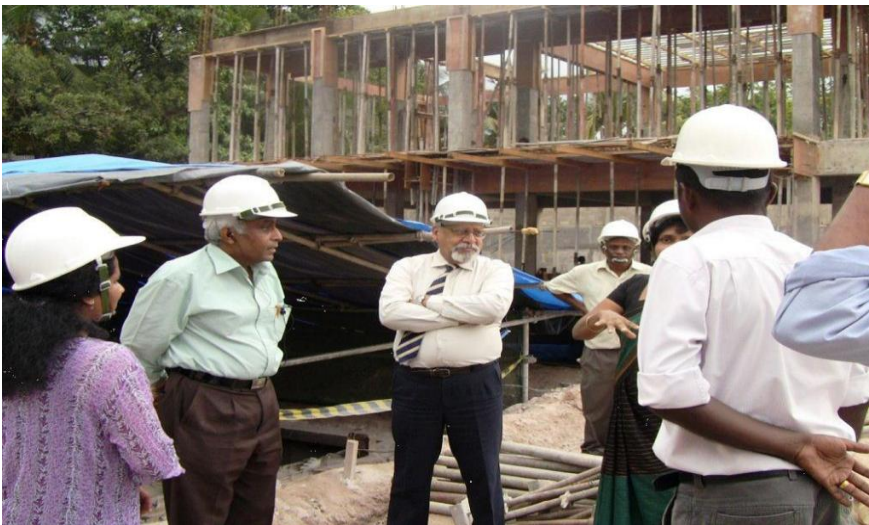
Fig No. 16: Construction of MGIF in Progress
