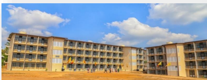
Four Storied 100 Rooms Hostel Building
