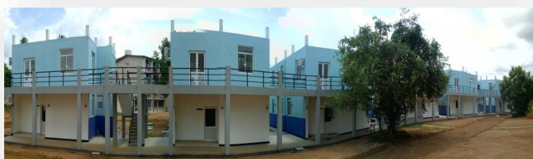
Laboratory Building to introduce Engineering Technology Degree Programme
