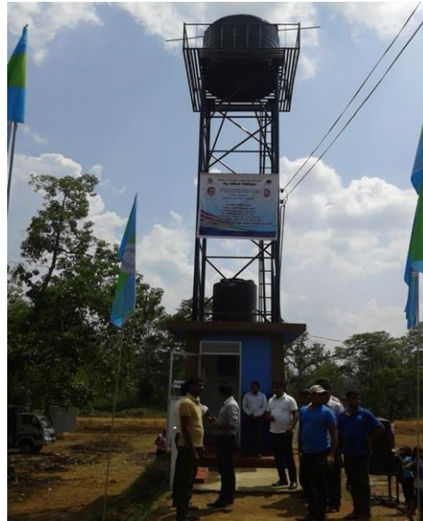
Fig 27: Thelulla water project
