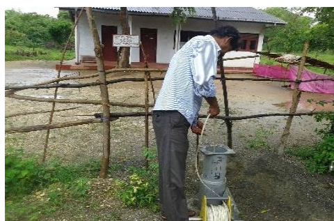
Fig8 :Rehabilitation of a hand pump
