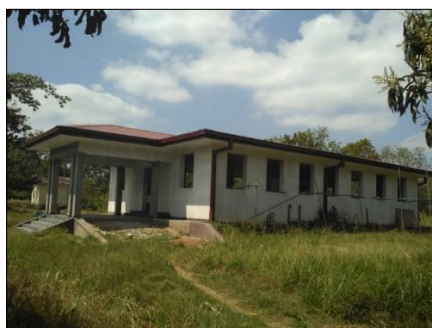
Fig 20 Newly constructing laboratory building at Provincial Office (NC/C)
