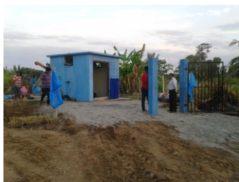
Figure 13: Construction of Pump House at Pallegama water supply scheme
