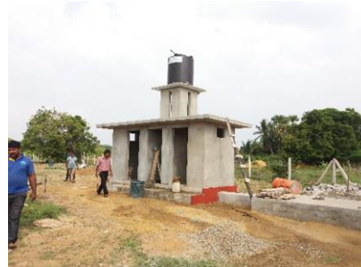
Fig 34 : Construction of Palai building
