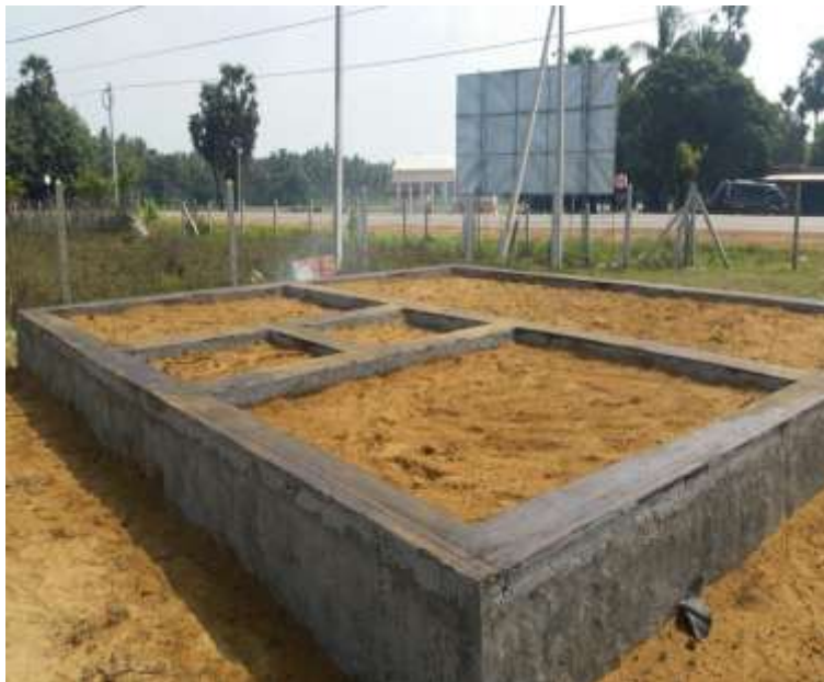
Fig 11: The initial construction stage of the proposed sub office for the North Provincial office at Pallai Land
