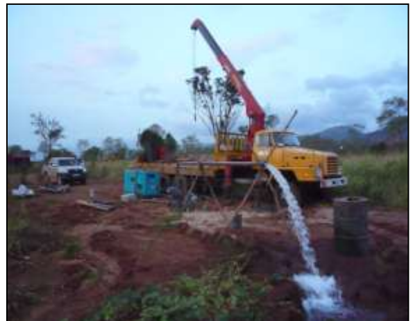
Conducting 24 hours pumping test
