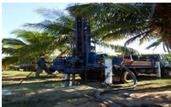
B) Geophysical Investigation at Vavuniya C) Tube Well Drilling at Kilinochchi
