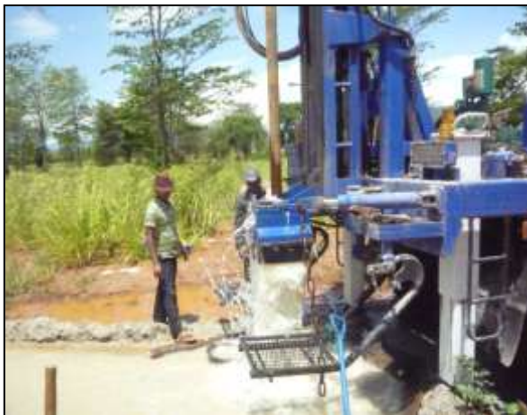
Tube Well Drilling
