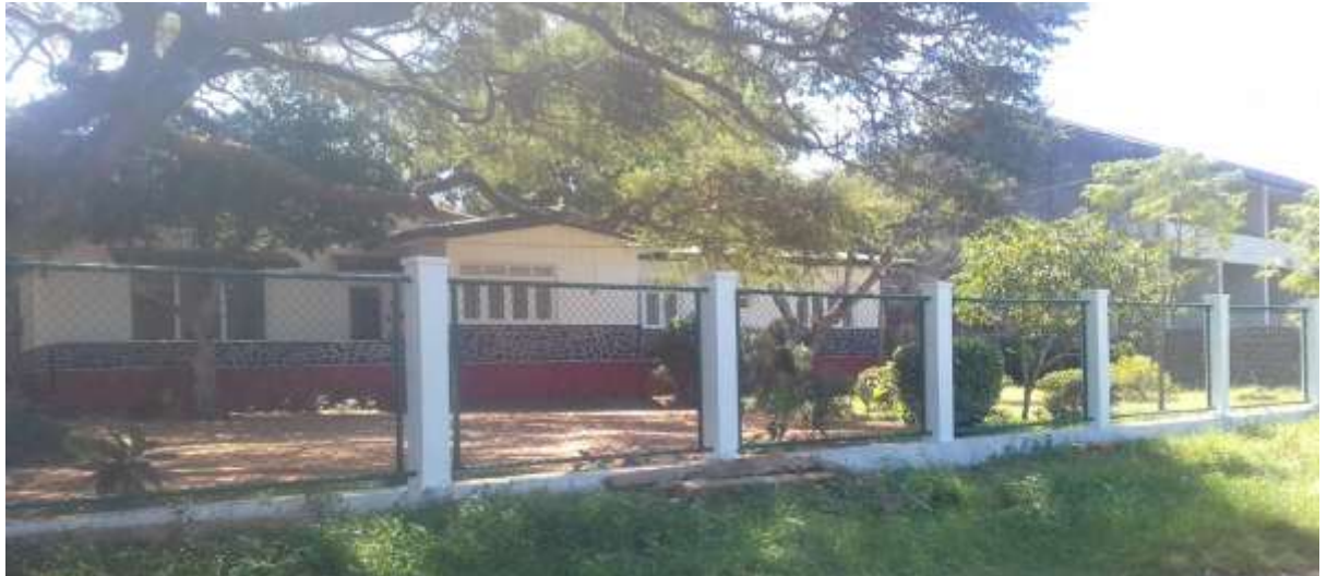
Photo 05: Repaired Circuit Bungalow at Anuradhapura
