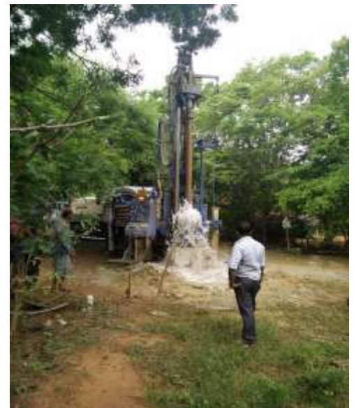
Figure 3.2 Drilling test well
