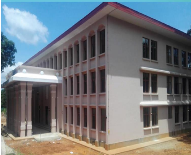
Construction of Geology Building, Faculty of Science
