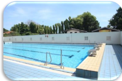
2. Sub Pool for training activities
