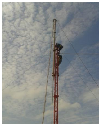
Pooneyrn wind measuring station – tower installation
