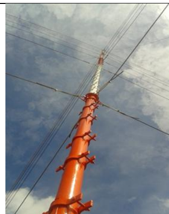
Mullipurama Wind Met-Mast after Major Maintenance
