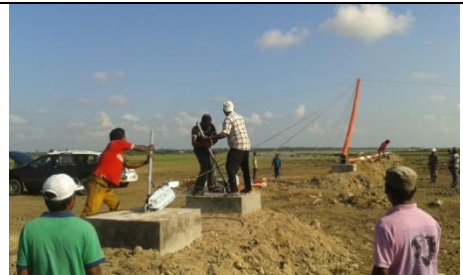
Kokilai wind measuring station – tower installation
