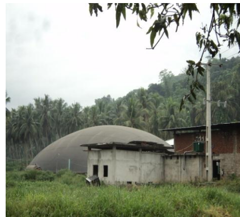
Grid connected Biogas Power Plant
