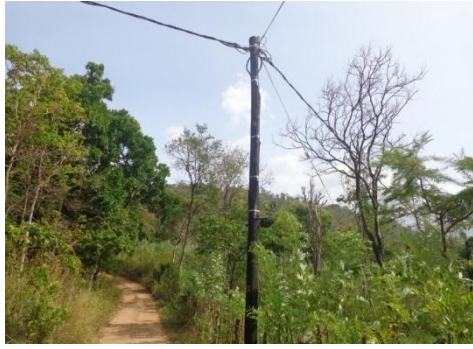
Electrification of 25 houses in Baduludena Village, Haputale
