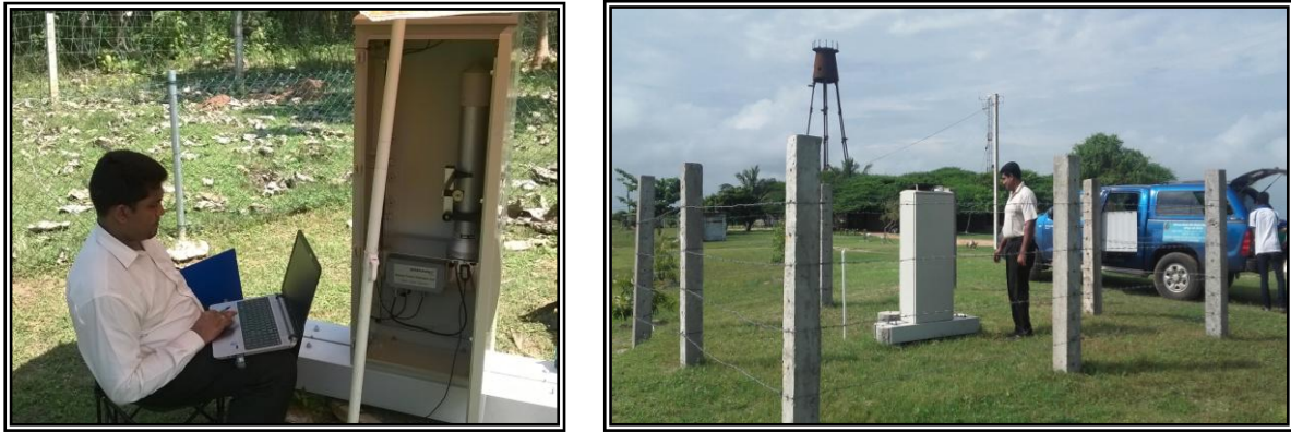
Figure 3: Remote monitoring Stations of Nuclear Disaster Early Warning System
