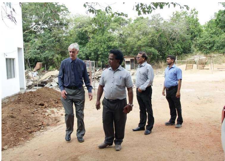
Observing the construction of the faculty building
