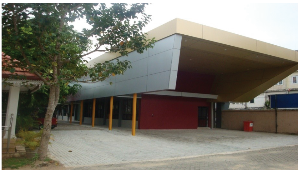
G.P.S. Control Room
