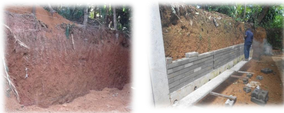
Construction of Post-tensioned Retaining Wall
