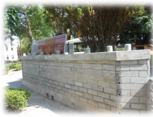
Post-tensioned Masonry Retaining Wall at Technology Park
