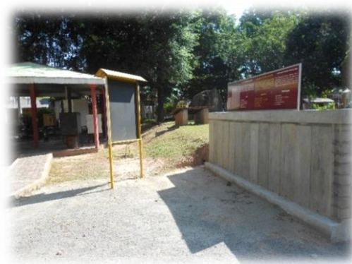
Pre-stressed Concrete Retaining Wall at Technology Park
