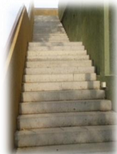
“L” shaped Prestressed Concrete Step
