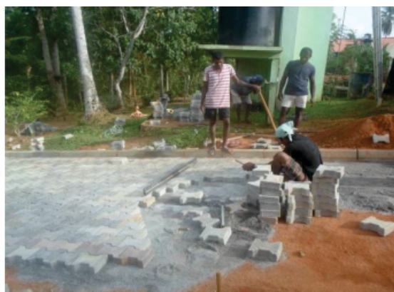
Inter lock stone laying – Navadigantha centre
