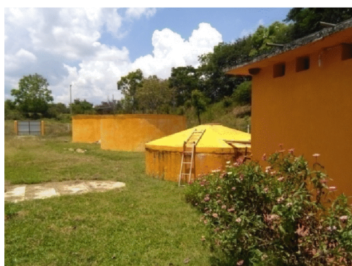
Community water purification units (sumps with two sand filters)
