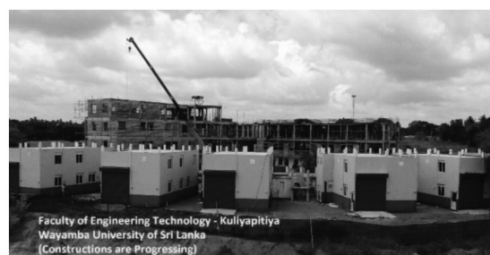
Construction of Laboratory building to introduce Engineering Technology degree programme – Wayamba University Kuliyaipitiya
