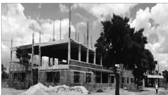
Building and other related structure for Engineering Technology and Bio System Technology -University of Jaffna
