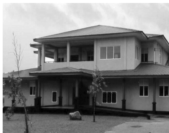
Construction of two storied dining hall & two storied multipurpose student center – Bhiksu University – TEC 213.4 Rs. Million
