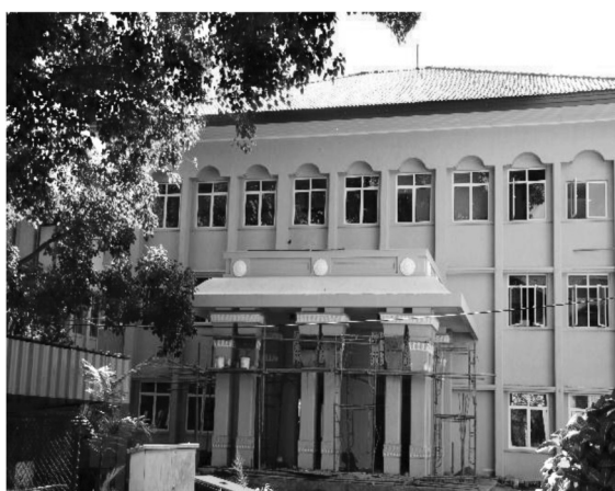
Building Complex of Postgraduate Institute of Science - Estimated Cost Rs.140 million
