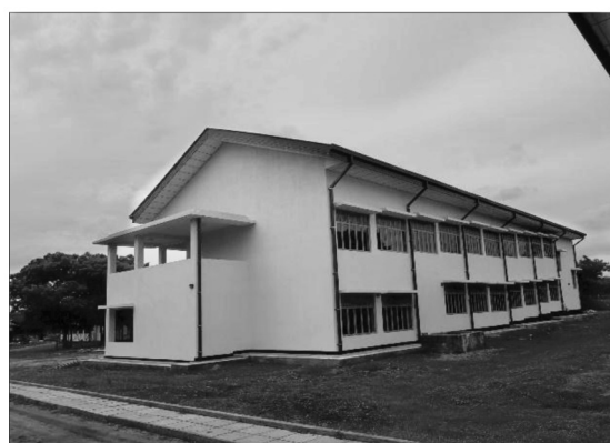
Construction of Secondary Pre Vocal Lecture Theatre- Vavuniya Campus
