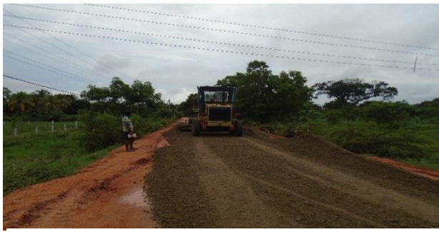
Construction of Kiriibbanwewa road
