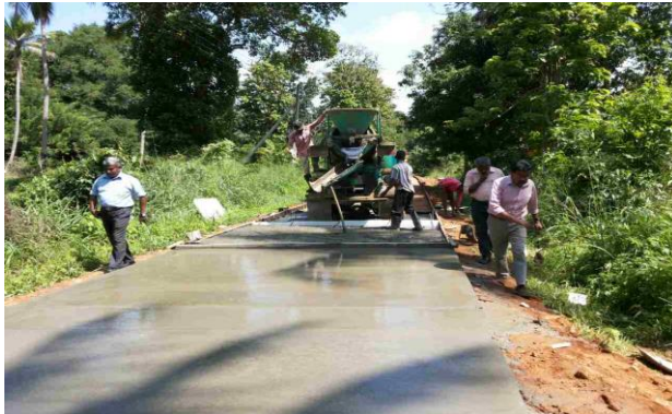
Construction of Dunukewela Road
