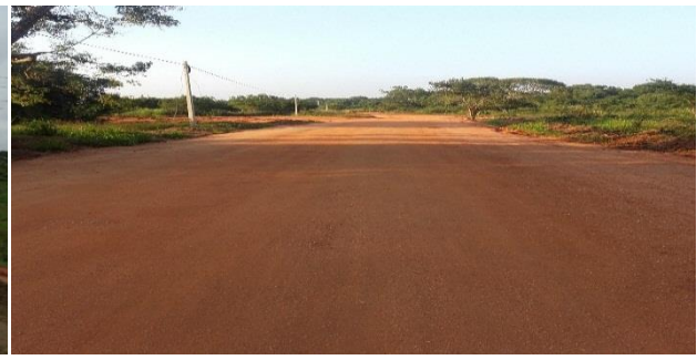
Construction of Gaiabapura –Nedunkani
