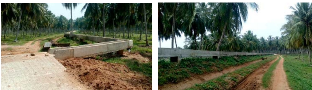
Newly constructed flood irrigation canals at Maduruoya Seed Garden
