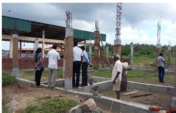
Construction of plastic waste recycling Model plant - Jaffna MC
