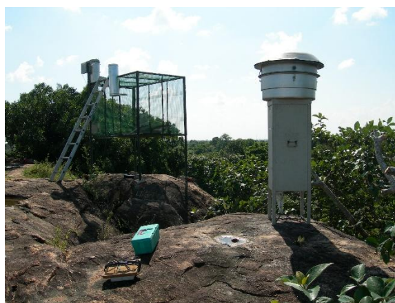
Instruments installed at Doramadalawa monitoring site
