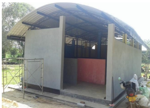
Recyclable waste storage center in Ippologama PS
