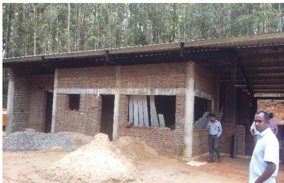
Construction of plastic waste recycling Model plant - Nuwara Eliya MC
