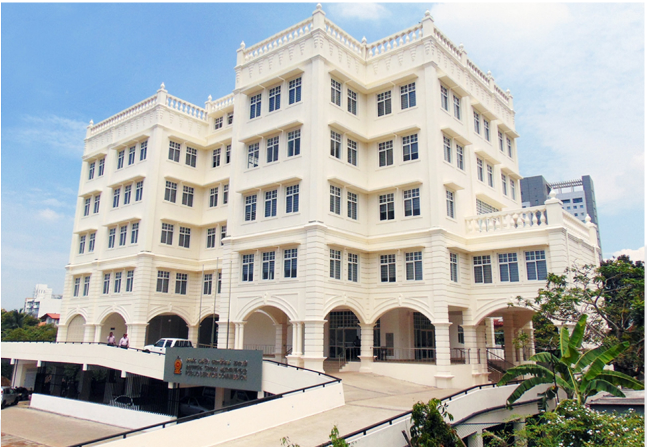
Public Service Commission Building at Battaramulla
