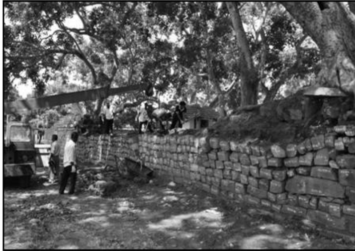
Conservation work in progress at the Monara Maligawa
