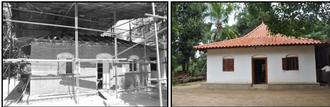
Pilawala Galedanda Mha Viharaya Before and after conservation
