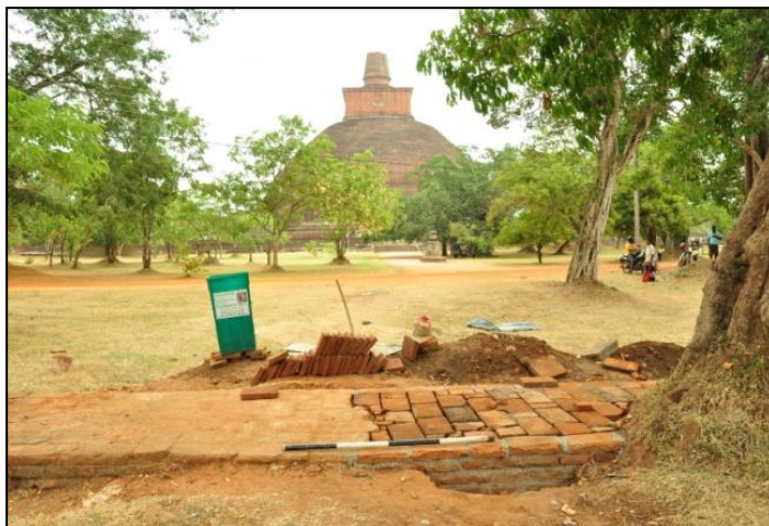
Conservation in progress in a bund at the Aramaya Complex
