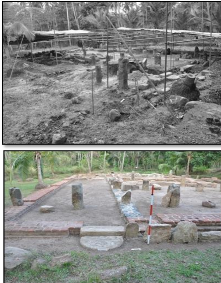
Building No.02 before and after conservat
