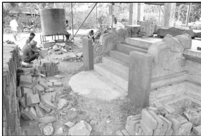
Conservation work in progress at the Monara Maligawa
