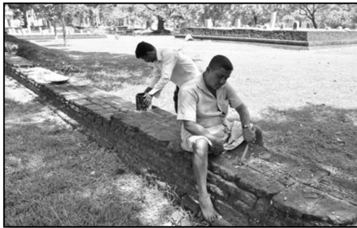
Filling of mortar joints
