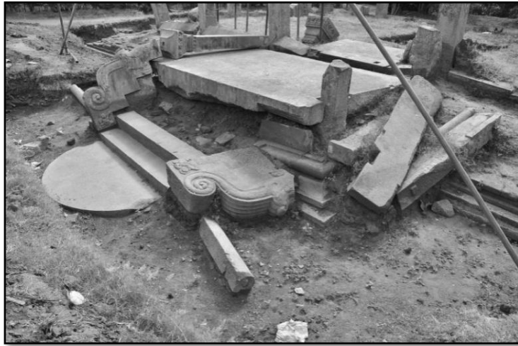
Conservation work in progress of the Monara Maligawa
