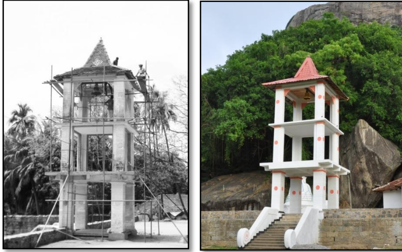
The Bell Post of the Yapahuwa Vehara before and after conservation.
