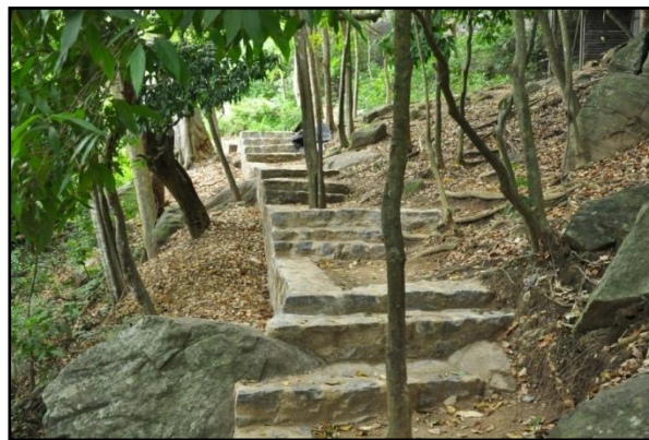
Conservation of stage II of the stairway
