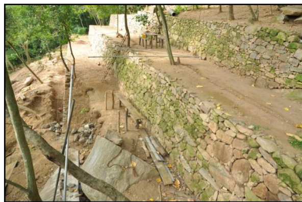
Conservation of retaining wall
