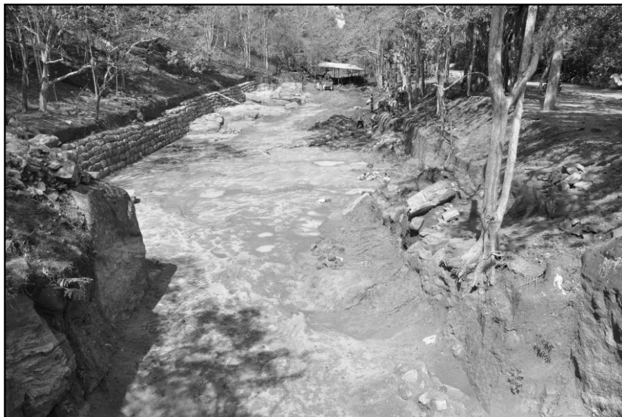
The site of the conservation at the end of the year.
