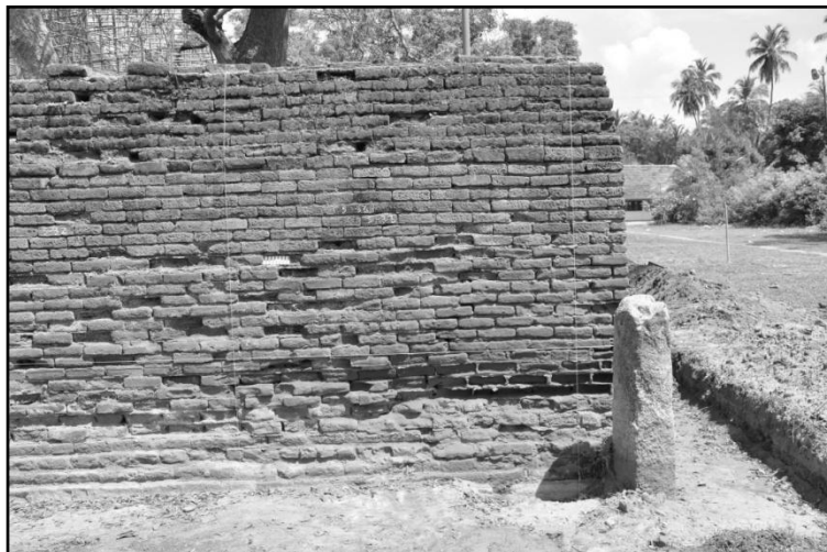
Sandagiri Stupa foundation.
