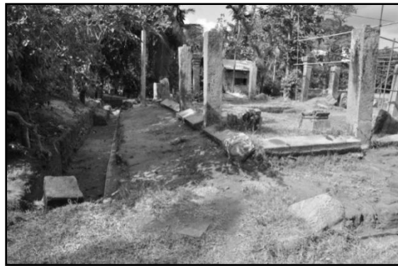
Construction work being carried out at the Peacock Mansion (Monara maligawa)
