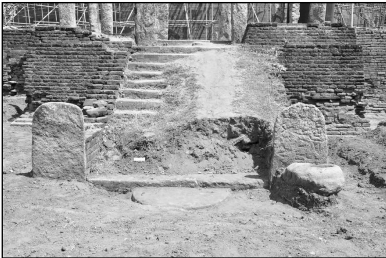
Sandagiri Stupa foundation.
