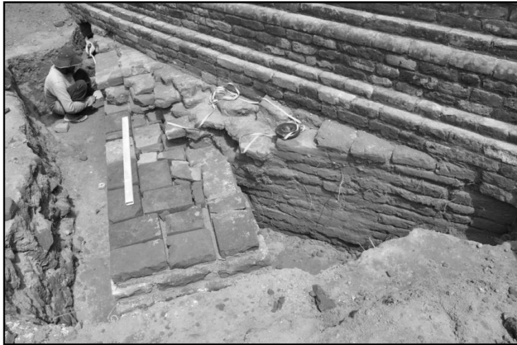
While excavation work was going on at Sandagiri Stupa foundation.
