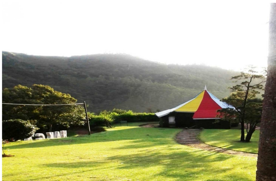
“Knox” Summer Hut – Following renovations
