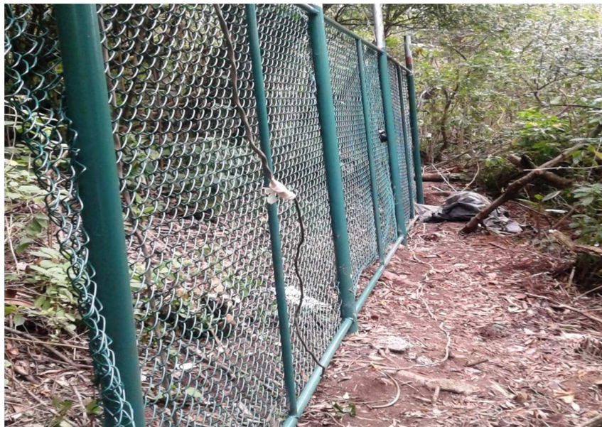
Chain Link Fence being renovated
