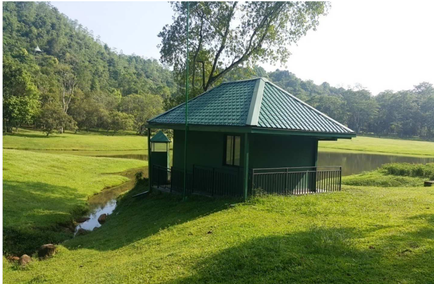
Boat yard erected at Avissawella Botanical Garden
