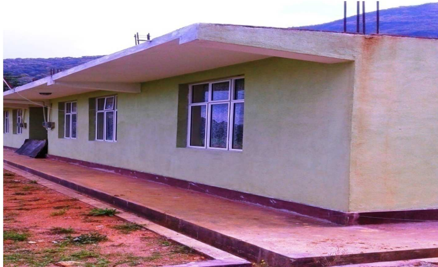
4 unit new official quarters being constructed
