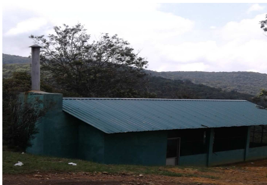
The new waste management building
