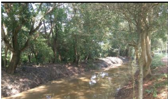
Drainage Improvement work in Natha Ela at Dippitigoda – Kelaniya
