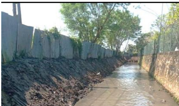
Drainage Improvement works at Wedhamulla connection canal
