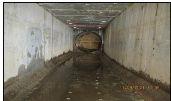
New Mutwal Tunnel
