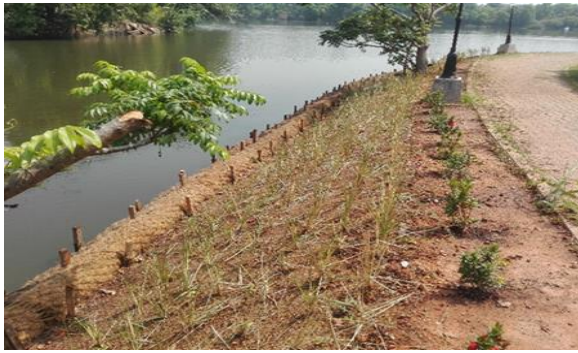
Figure 1 : Just after finishing the restoration process
