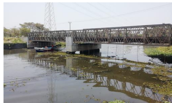
40m span Bridge at Karadiyana
