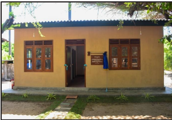
ND Nariwilamkulam at SLNS Pussadewa
