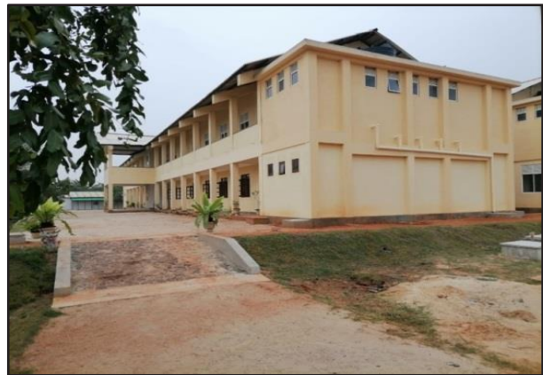
J/S Accommodation Building
