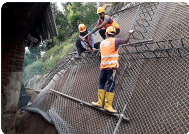
Mitigation work at NIFS Kandy
