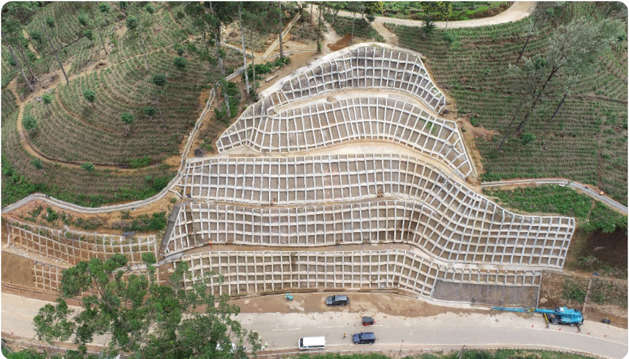
Landslide Mitigation Completed site - Site No: 148 Nallathanniya (Package 09)
