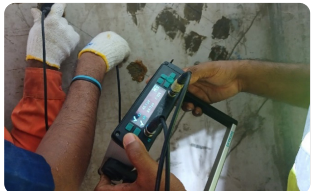
Non-destructive testing on the diaphragm wall
