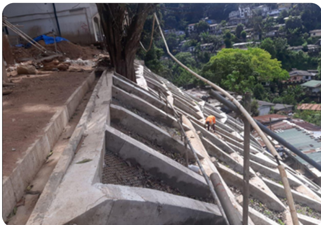
Slope Stabilization Works
