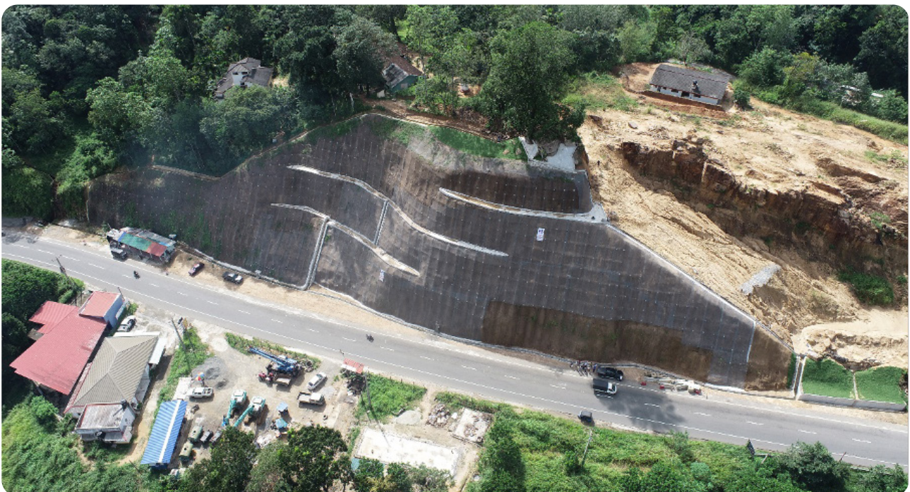
Landslide Mitigation Completed Site - Site No: 011 Kegalle By-pass Road (Package 04C)
