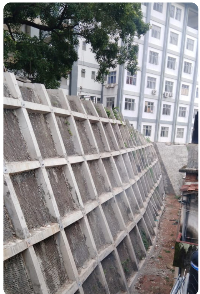
Landslide Mitigation Project at University of Kelaniya
