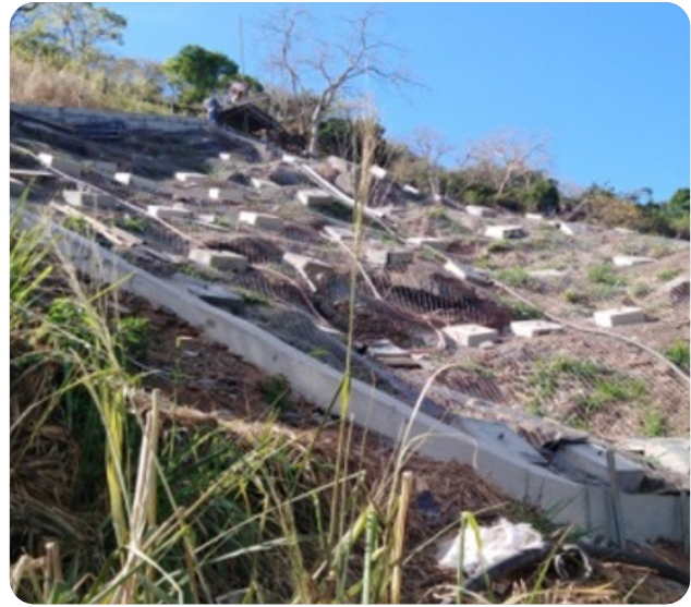
Landslide Mitigation Project at Malapattawa
