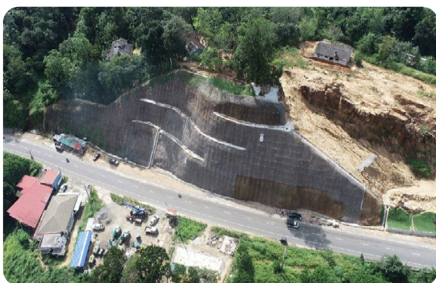
Mitigation work at Kegalle bypass road under RLVMMMP
