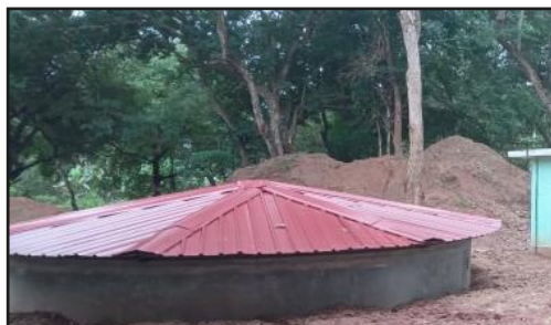
Constructed Agro well at MTC
