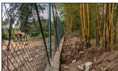
Renovated boundary fence at GMPG
