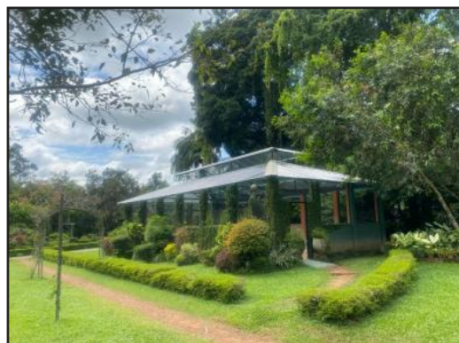
Repaired plant house at GBG
