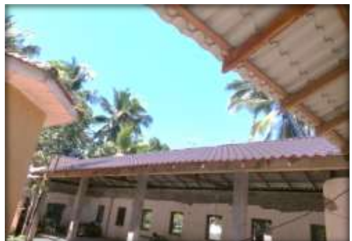
Renovating roof of the Sudarshanarama Viharaya in Biyagama
