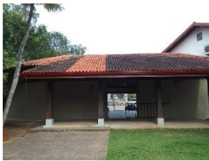
Renovation of the roof
