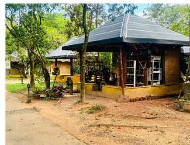
Renovation of the stalls
