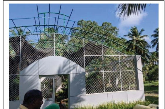
The roof of the renovated plant house
