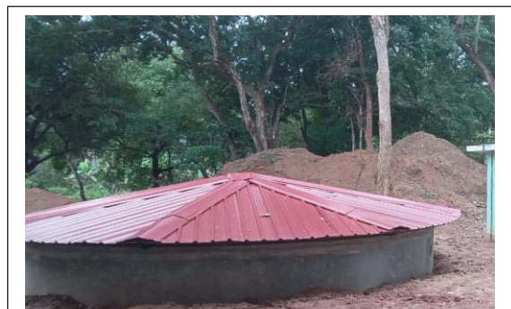
Well under construction
