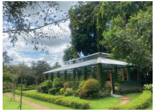
The roof of the renovated greenhouse
