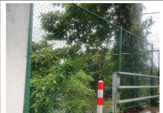
Completed Installation of the new entrance gate
