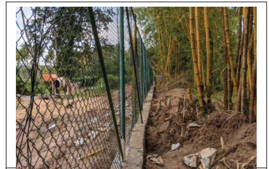
Newly constructed chain link fence
