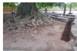
Conservation of damaged parts of Seruwila Stupa Courtyard
