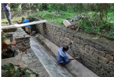
Conservation of outer walls
