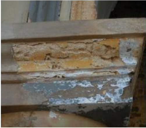
Before the conservation of the plaster of the Duwa Sindrathi Church at Negombo, degraded due to salt
