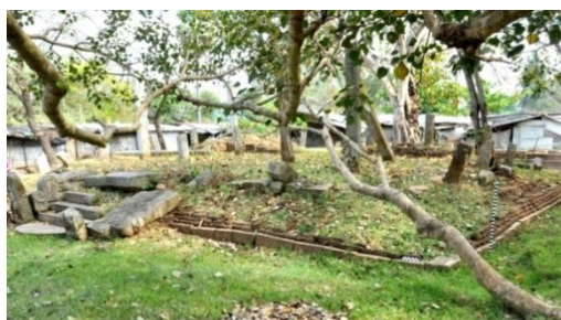
Tuparama Building No. 60 Before conservation
