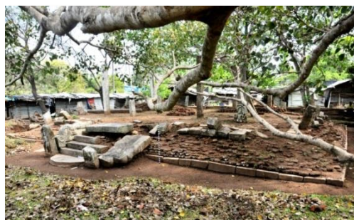
Tuparama Building No. 60 After conservation
