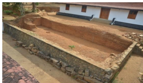
After the excavation of the front of the new Museum
