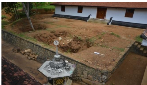
Before the excavation of the front of the new Museum
