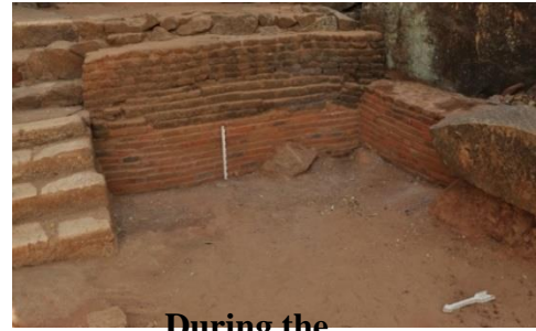
During the excavation of the channel around the Seethala Maligawa at the right side
