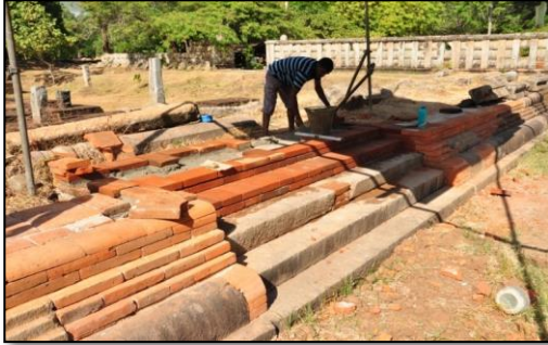
During the conservation of the Bodhigara building
