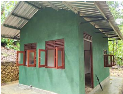
Figure 2-12: Construction of a new ticket counter at Andahalena Ella
