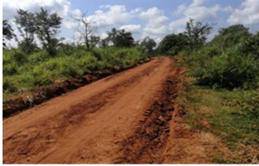
Figure 2-9: Laying and pressing of gravel on 13.5km portion of safari jeep road located within Hurulu eco park
