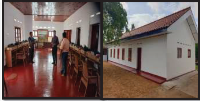
Renovation of DhathuMandira and library building of the Thissamaharama Raja MahaViharaya
