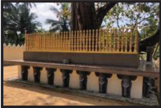
Completion of renovation activities of Bodhi Prakara in Keragala Raja MahaViharaya
