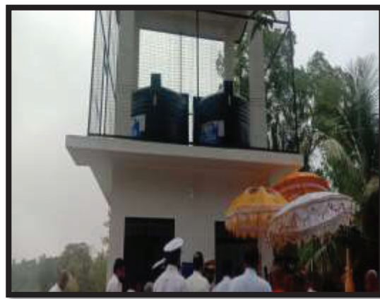
Installing water filter system of Thooparama Raja MahaViharaya
