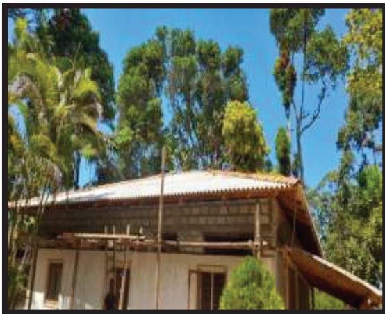
Sri Sudarshana Buddhist Center Repairing the monastery
