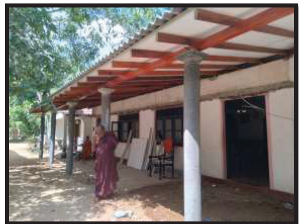
Nawagamuwa Purana Viharaya Remaining construction of the monastery
