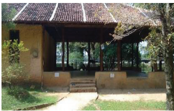
Renovation of outdoor theatres
