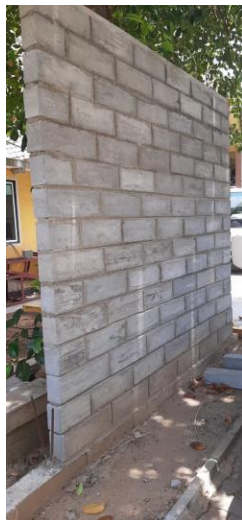
Wall constructed with light weight blocks
