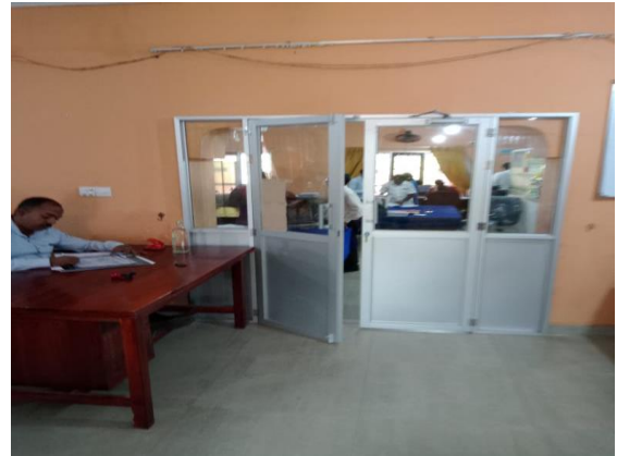
Trincomalee Land Registrar Office - Renovation of building
