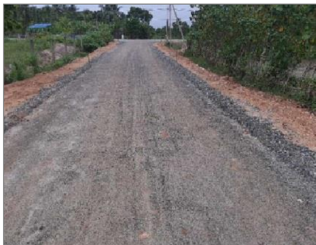
DGAB work at NMU037 at ch. 01+700
