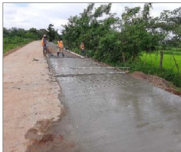
Construction of rigid pavement on NMU 070 at ch.04+350
