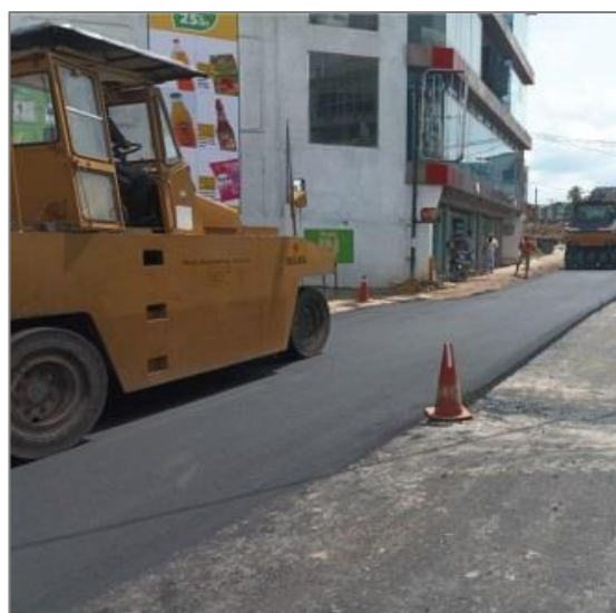
Asphalt binder laying at ch. 90+870 (LHS)
