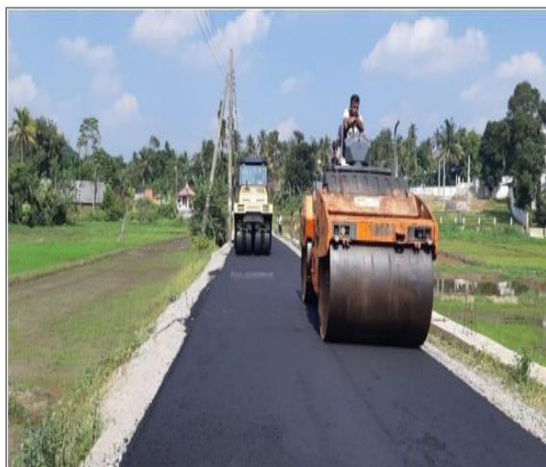
Asphalt Concrete Surfacing at WCO 186
