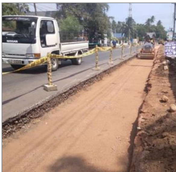
Sub base compaction at ch. 50+000 – 50+300 (RHS)
