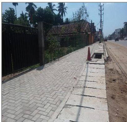
Drain and foot walk construction at Ch.7+000
