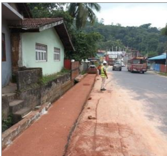
Sub base construction for widening at ch. 93+720 (RHS)
