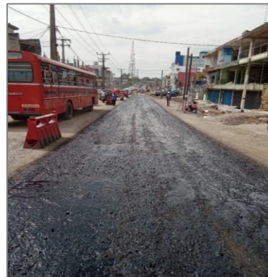
ABC Priming Work at Ch. 2+800 LHS -
