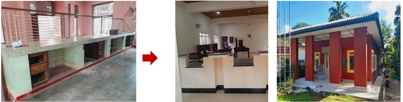
Figure 2.25:- Post Office, Wasalakotte
