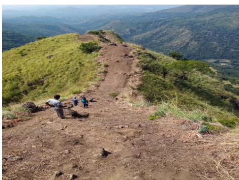
Conducting road construction activities
