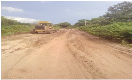
Reconstruction of internal roads
