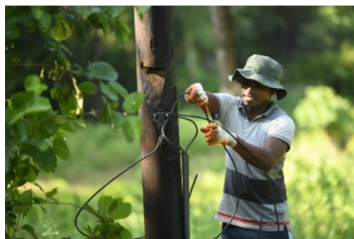
Renovation of electric fences
