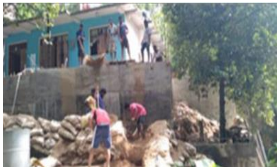
Multi-purpose Development Assistants helping to renovate a house affected to landslide - Udunuwara
